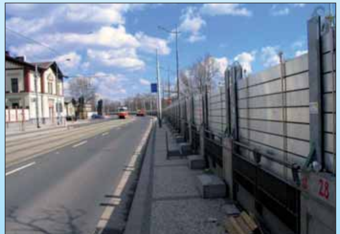
Fig. 4.21 Mobile Flood Barriers in Prague – Holešovice (Source: VRV a. s.).
