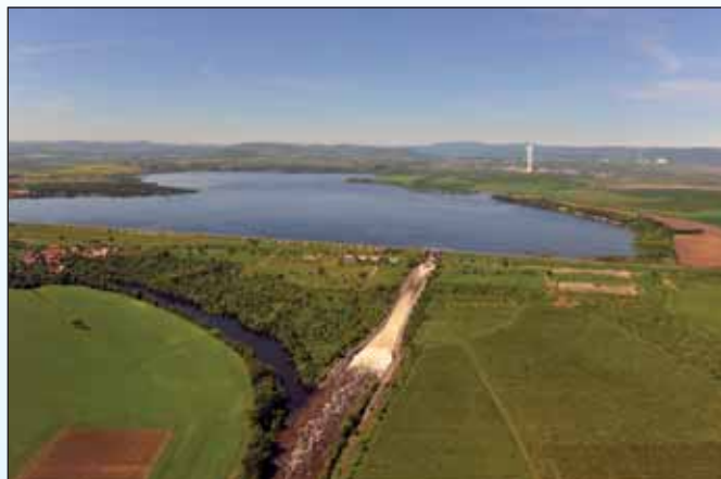
Fig. 4.11 Nechranice Reservoir – Aerial View of 5 June 2013 (Source: Povodí Ohře, s. p.).
