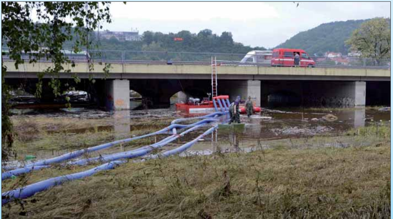
Fig 5.1 Intervention of Firefighters in Prague-Chuchle (Source: Prague - Velká Chuchle Municipality).
