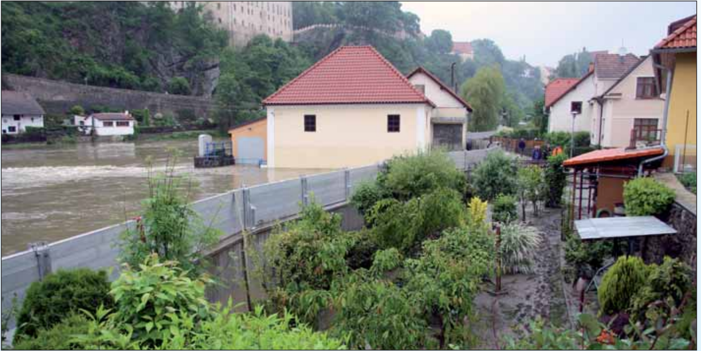
Fig. 4.17 Mobile Flood Barriers along Lužnice River in Bechyně (Source: VRV a. s.).
