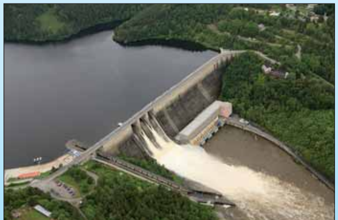
Fig. 4.4 Orlík Reservoir – Aerial View on 4 June 2013 (Source: Povodí Vltavy, s. p.).
