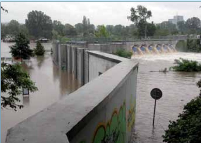
Fig. 4.20 Prague-Libeň – Pumping of Rokytká Stream Water to Vltava River (Source: VRV a. s.).
