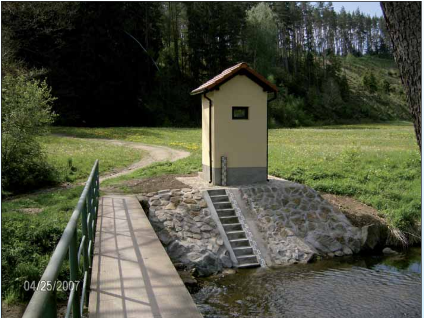
Fig. 7.3 Reconstructed Station Slovénice on the Chotýšanka Stream. The Station remained functional during the flood in June 2013 with the peak exceeding the 100-year flow rate.
