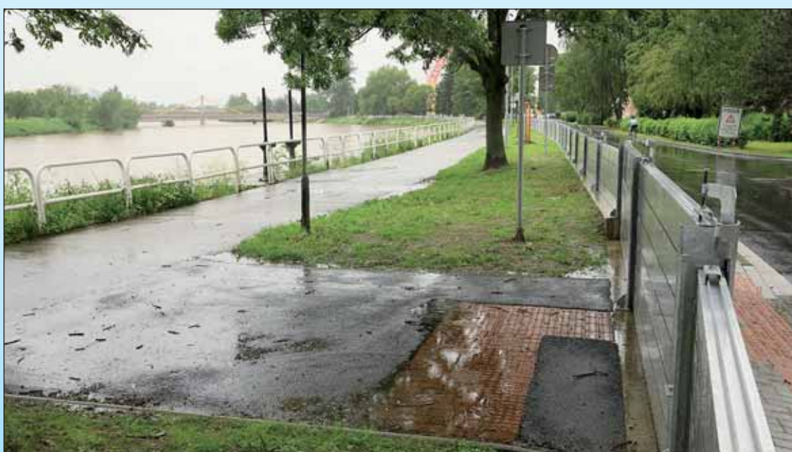
Obr. 4.16 Mobile Flood Control Barriers along the Vltava River in České Budějovice (Photo by Libor Sváček).
