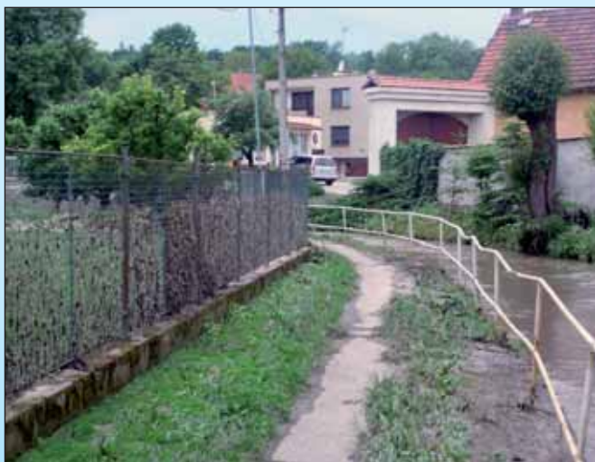
Fig. 2.3 Traces of Peak Level after Flood in Běloky on Dolanský Stream. (Source: official website of the village of Běloky).
