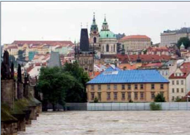
Fig. 4.18 Mobile Flood Barriers in Prague downstream of Charles Bridge (Photo by Jan Kubát).
