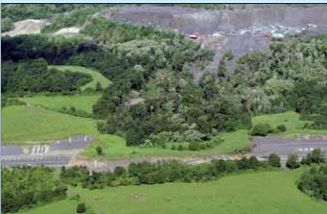
Fig. 5.6 Aerial View of Dobkovičky Landslide on 11 June 2013 (Source: ČGS).
