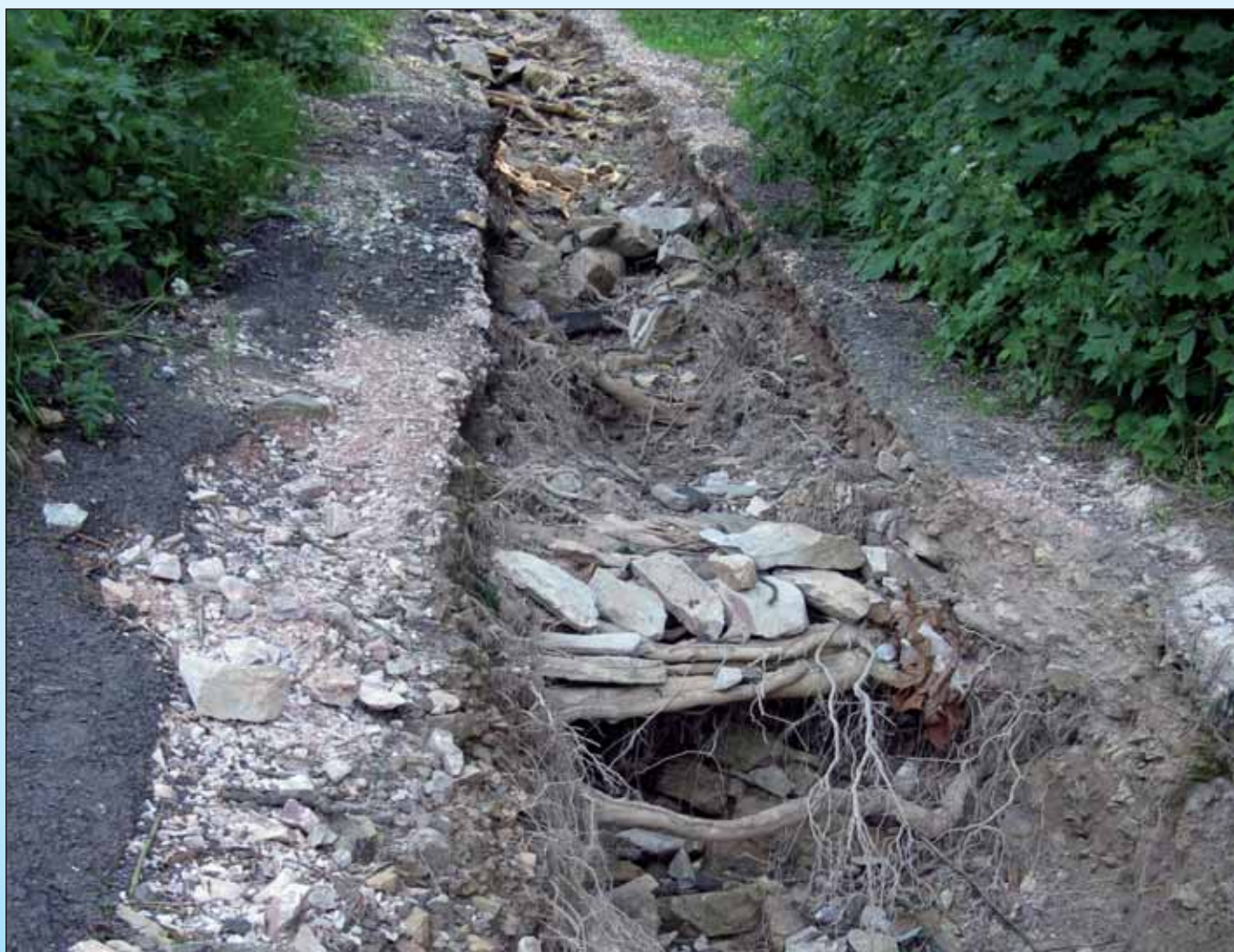
Obr. 2.16 Fluvial Erosion on the Hiking Trail above Horní Maršov (photo by Radovan Tyl).
