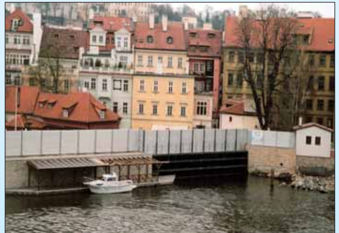
Fig. 4.19 Closed Outlet of Čertovka Channel in Prague (Source: VRV a. s.).
