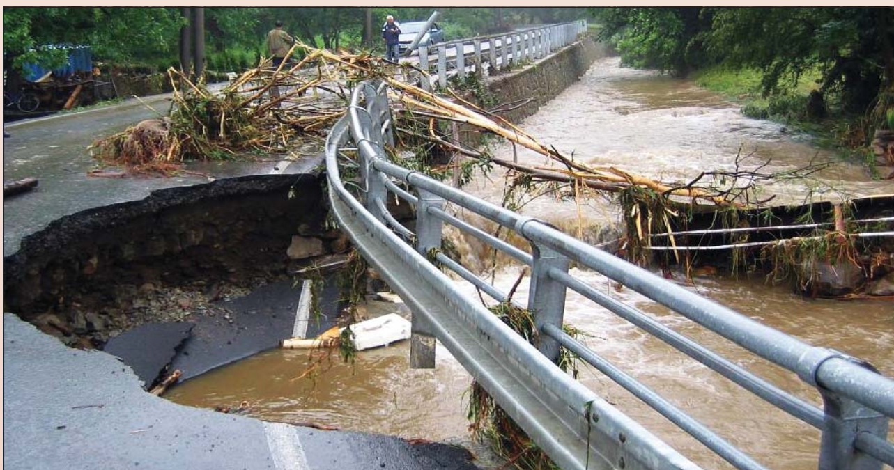
Obr. 6 Zničená komunikace v obci Žulová-Tomíkovice. Fig. 6. Destroyed road in the village of Žulová-Tomíkovice.
