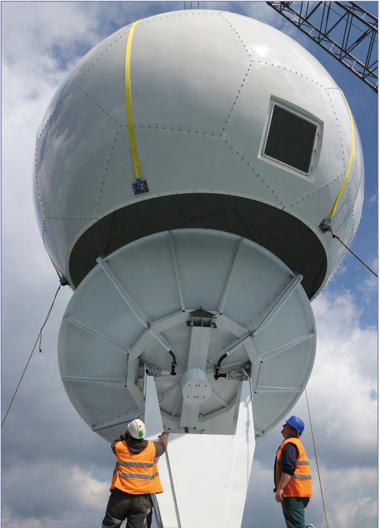
Instalace nové kopule antény na radarovou věž radaru Brdy. Installation of the new antenna dome on the Brdy radar tower.
